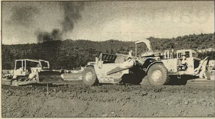
Approximately 52,000 cubic yards of soil were moved to level the sight that would become the New Fairchild Medical Center.
