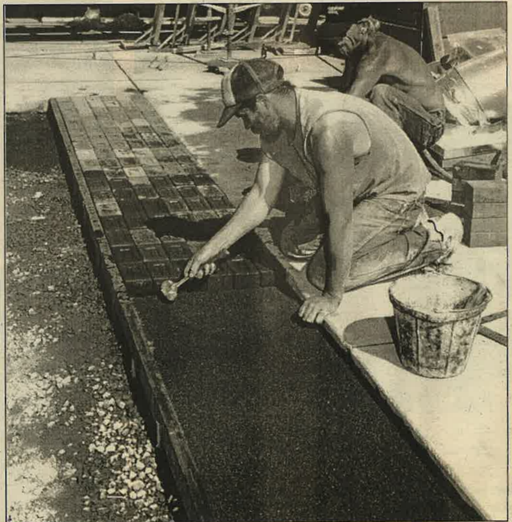
A worker begins laying the donor bricks. Note the top grooves in the bricks. This is where the personalized plaques will be placed. The bricks run along both sides of the front of the hospital and then up to the door.
