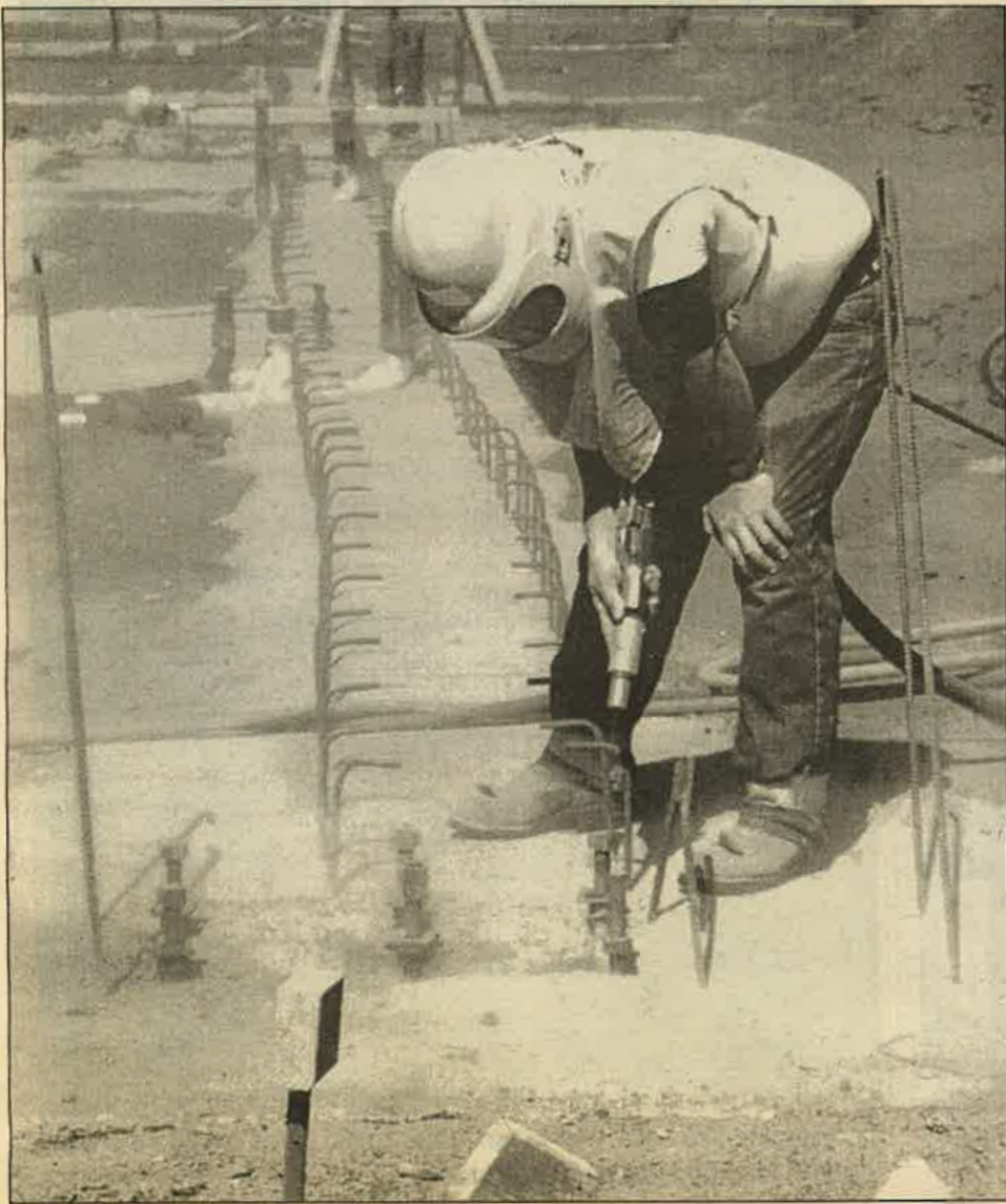
Above, steel workers congratulate one another upon completion of the structural framework for a job finished without any accidents or injuries. This "topping off" ceremony is a tradition among steel workers. At left, Ray Hjertager of Etna sandblasts a newly poured footing to allow the floor slab to bond securely with the footing. Below, steel workers hold on with their feet and legs while applying bracing between the large steel beams.
