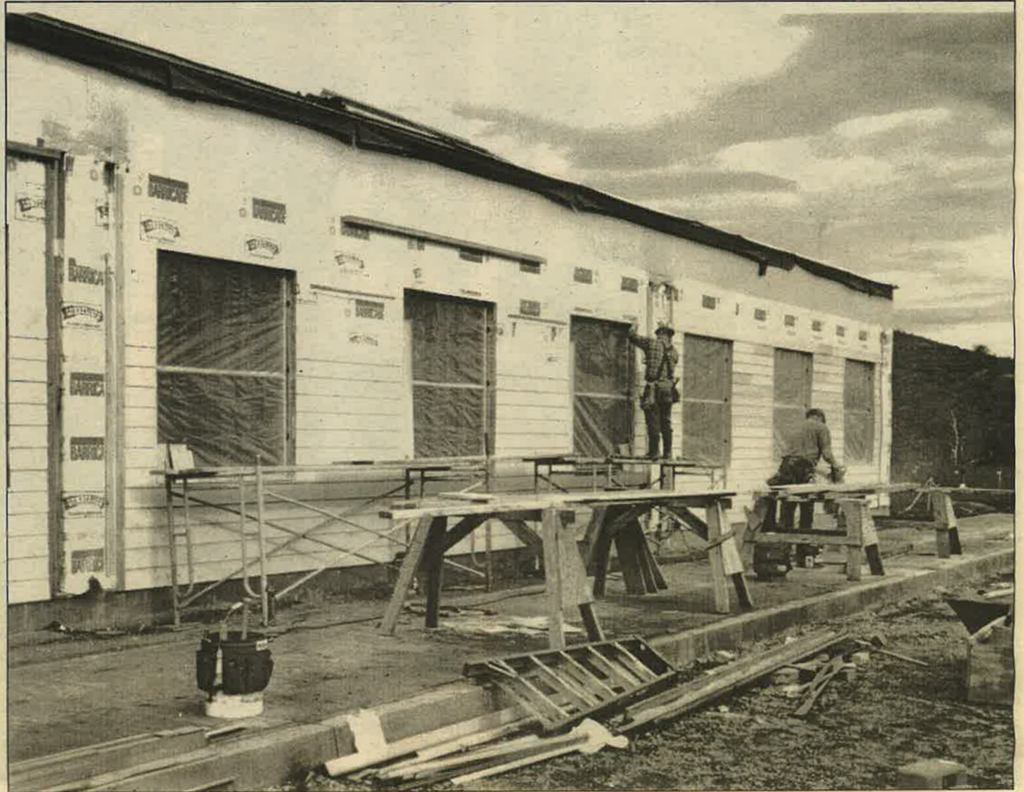
Phil Laubacher (right) of Big Springs installs siding over vapor barriers on the outside of the facility.
