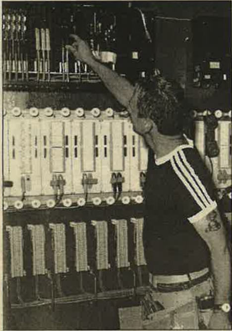
Ron Toth (above) of Executone installs the telephone and data circuits.
